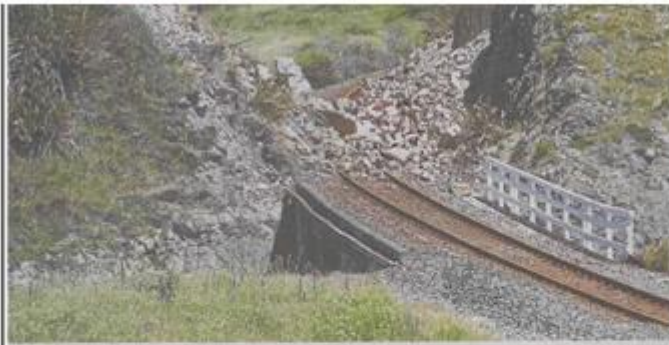
Fibre optic sensors could have provided more immediate warning of damage to this rail line north of Kalkoura.
